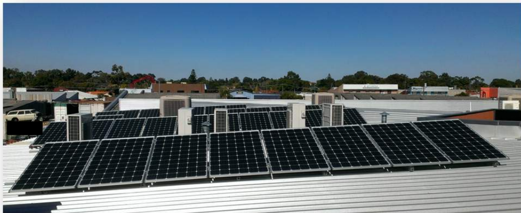
The Roof of NL-Tec's Office and Warehouse Building
